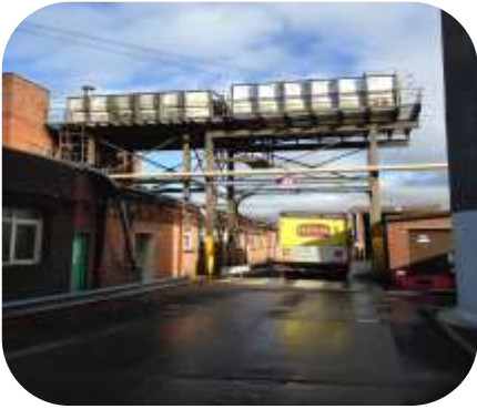
Structural steel underneath a water tank abrasive blast cleaned and coated with Resichem 501 CRSG
