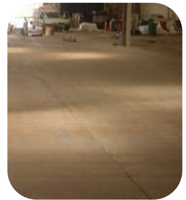
Concrete surface primed using Resichem 503 SPEP prior to application of Resichem 501 CRSG
