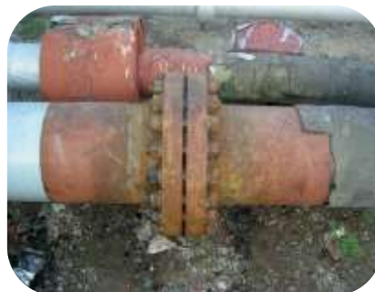
Badly corroded pipe surfaces were hydro-blasted at a European refinery and coated with 2 x coats of Resichem 501 CRSG to give long term protection against CUI
