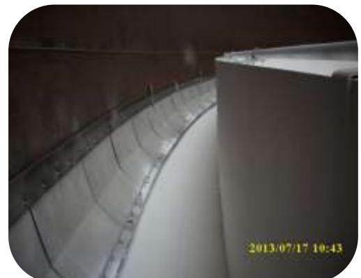
Floating roof on crude oil tank hydro blasted at 1000psi, primed using 506 Aluprime and over coated with 554 RB membrane
