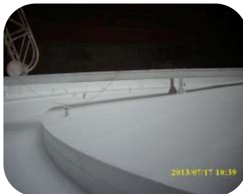
Floating roof on crude oil tank hydro blasted at 1000psi, primed using 506 Aluprime and over coated with 554 RB membrane
