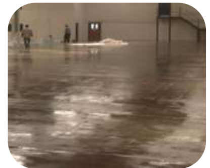
Concrete surface on a chemical containment area was mechanically abraded and sealed with Resichem 503 SPEP prior to being over coated with Resichem 501 CRSG
